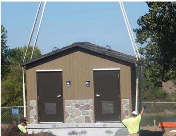
*A crane sets the restroom building into place.*
